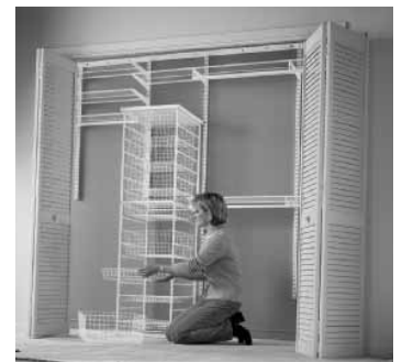
Position the Drawer Unit in the closet.
