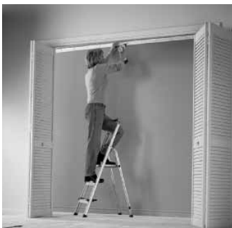
Place the Hang Track at ceiling height or door height.
